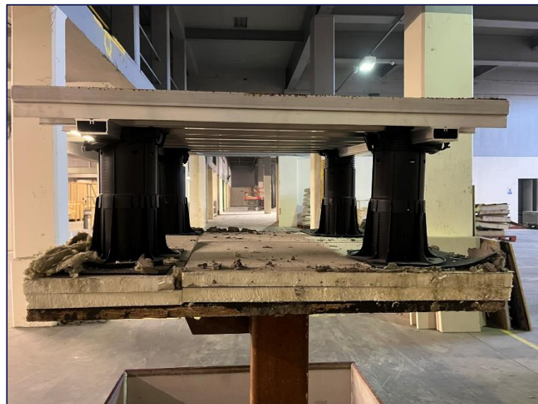
Figure 15: Damage investigation – Sample G – Side view.
